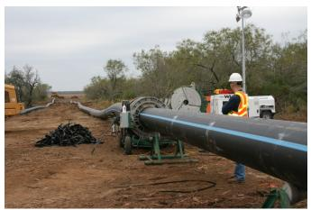
"Quality control and on-site testing were important issues for SAWS," said Radoszewski, "and would have been very costly to do for coated steel pipe. HDPE proved to be a leak-free material, with no cathodic protection required, leading to lower maintenance costs, which was critical given the remote location of the
